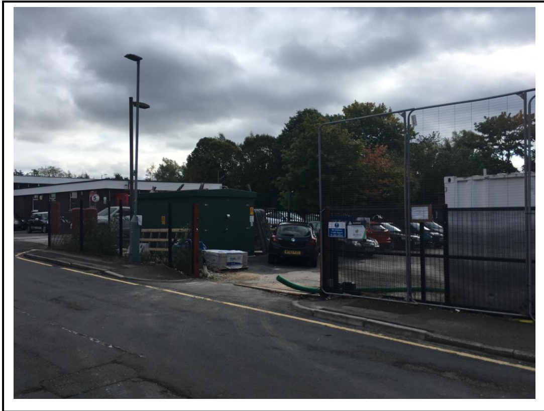
Substation (in situ)
